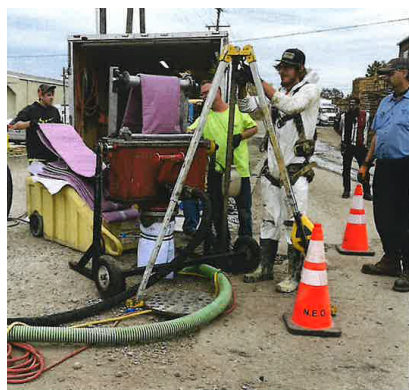
Crew lining broken sanitary main
