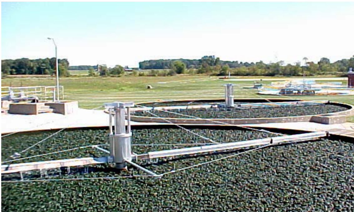
68 Foot Trickling Filters
